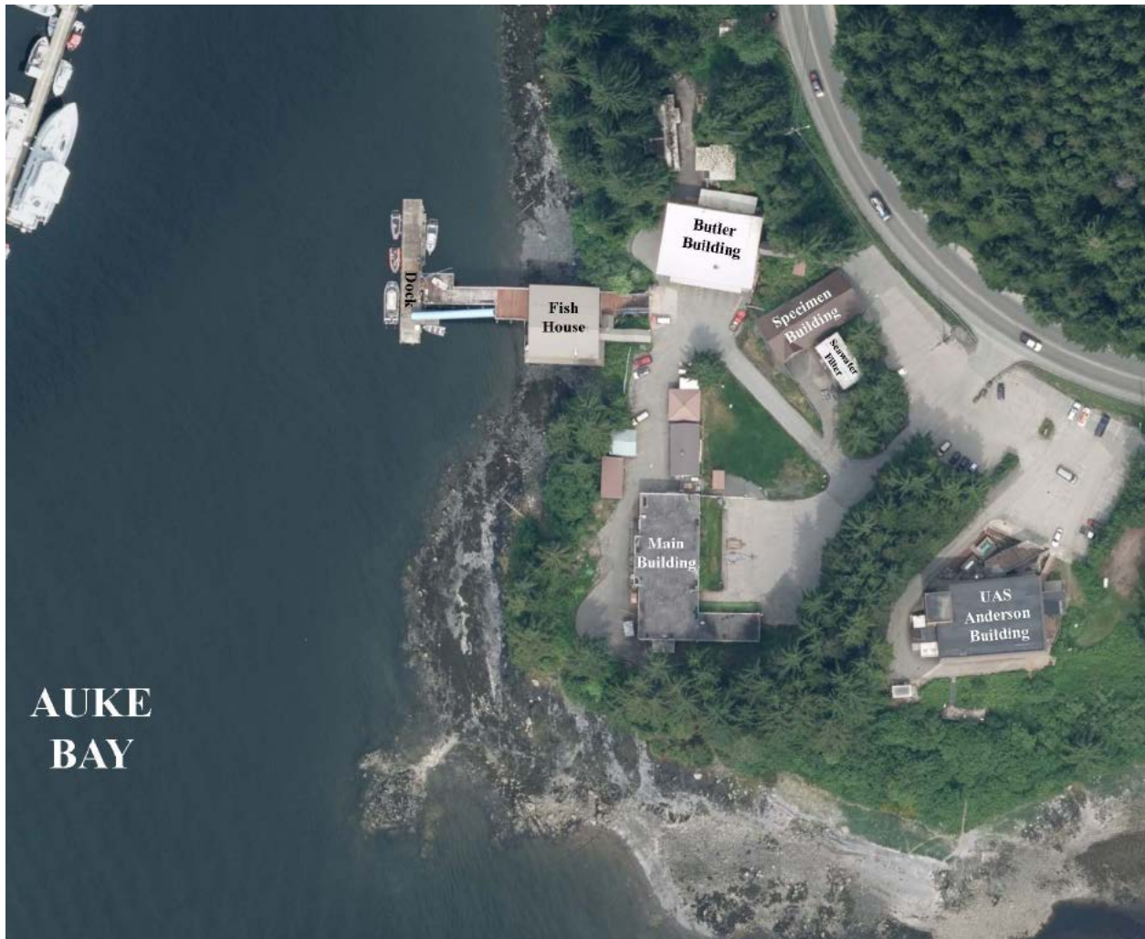
Aerial view of the NOAA Auke Bay Marine Station property and the adjoining University of Alaska Southeast Anderson Building
