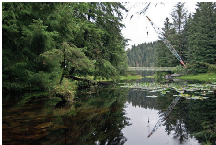
Bridge over Auke Lake outlet
