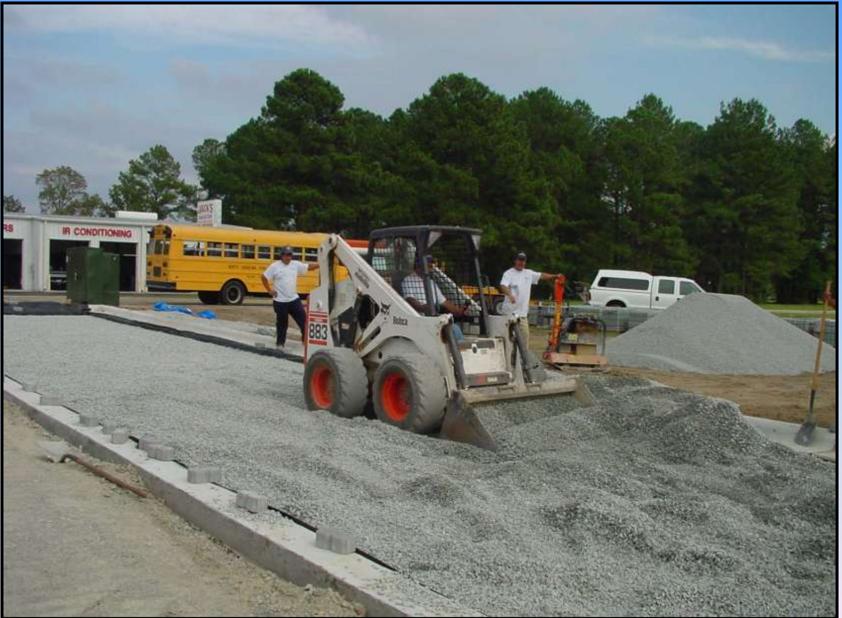
Final grading of base material
